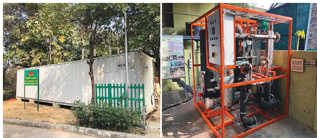
View of the containerized biogas plant and chiller system at biogas plant research facility of TERI
